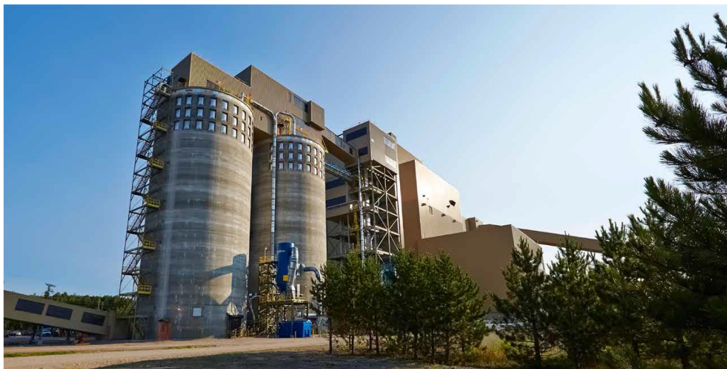
Figure 6.2 Two new silos were constructed at Atikokan during the conversion to biomass. Each is 44 meters tall, and holds approximately 5,000 tonnes of wood pellets.
