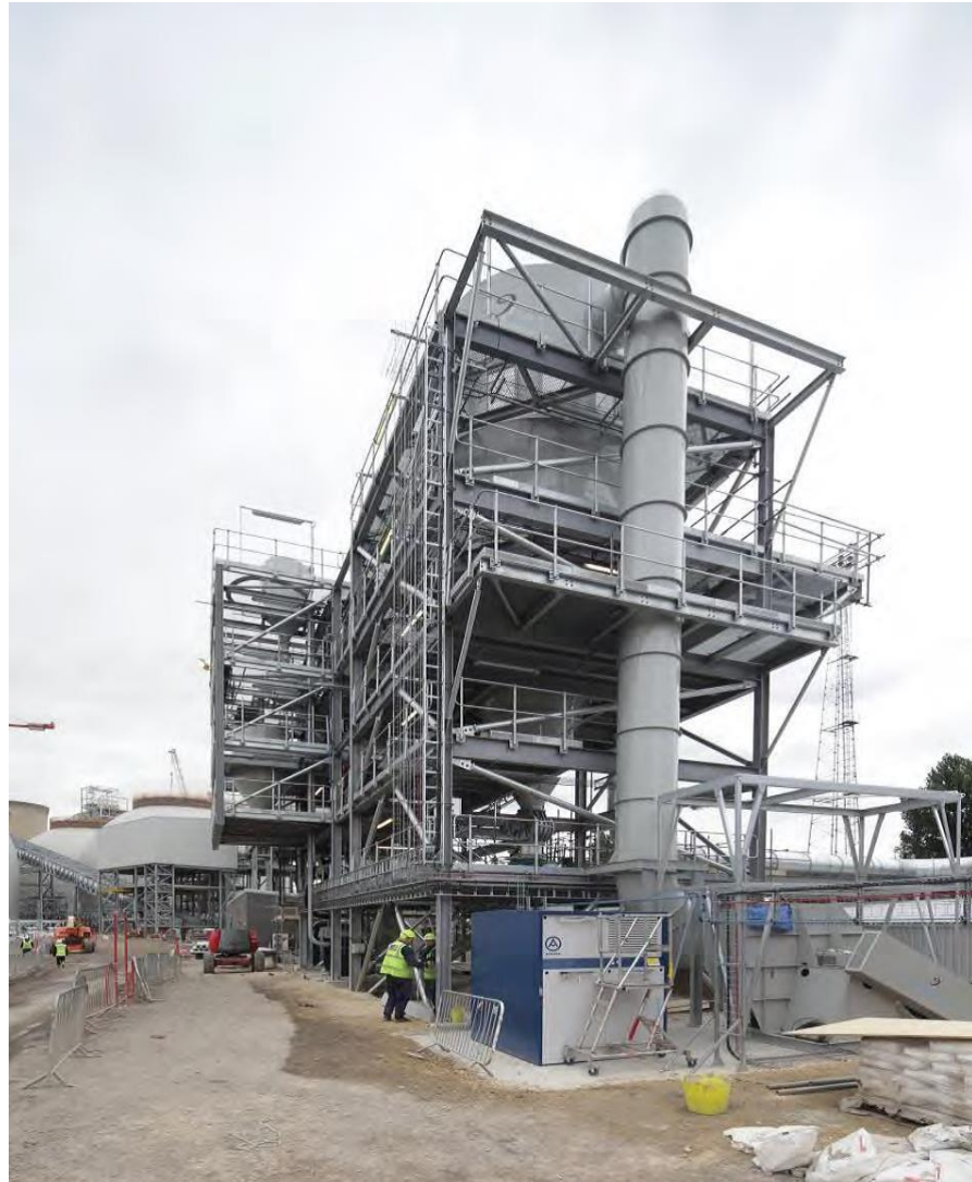
Figure 5.3 One of the large dust extraction systems
