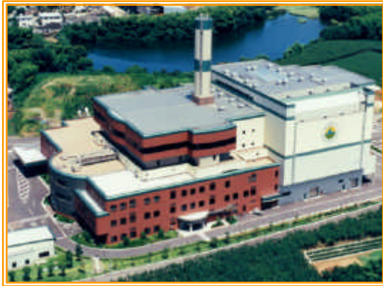
For: Yame Seibu Regional Administrative Association 110 ton/day 2 trains Start Const. 1997 *Completed March 2000
