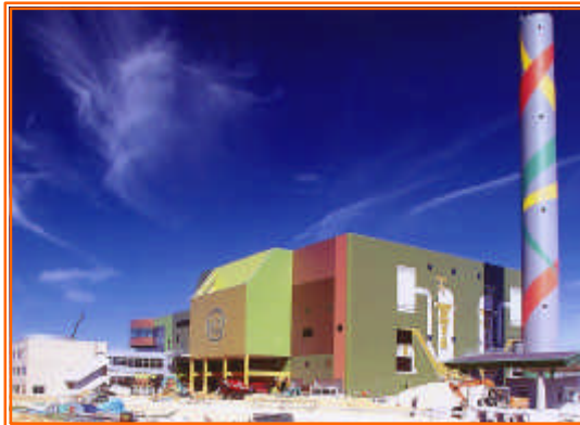
For: Koga City and One City, Four Towns' Waste Disposal Cooperative 130 ton/day 2 trains Start Const. 2000 *Completed March 2003
