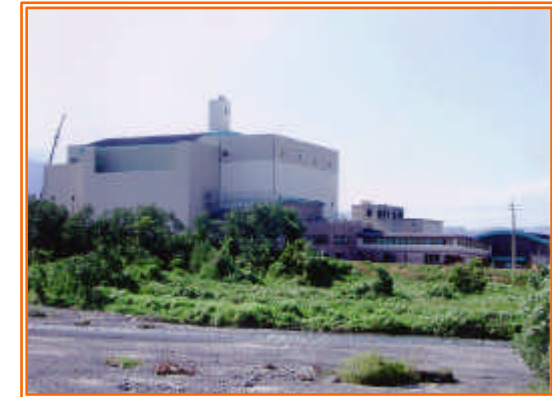
For: Kyohoku Regional Administrative Association 80 ton/day 2 trains Start Const. 2001 * Completed March 2003
