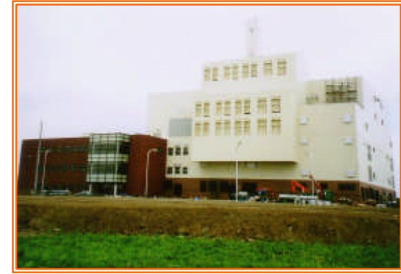
For: Ebetsu City 70 ton/day 2 trains Start Const. 2000 *Completed Nov. 2002
