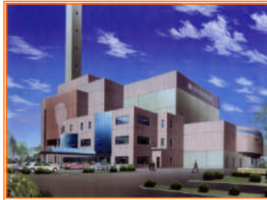
Owner: Nishi Iburi Regional Union Operator: Nishi Iburi Kankyo Co. Ltd 105 ton/day 2 trains Start Const. 2001 *Completed March 2003
