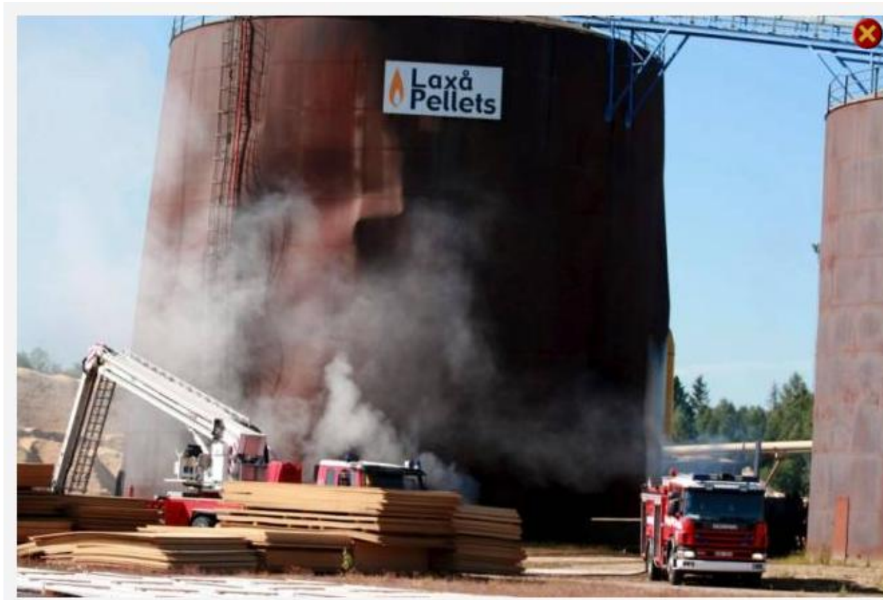
Explosion during fire fighting damaged the silo structure
