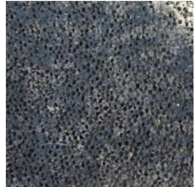
Foam ceramic after 2 heating seasons Approx. 550 batches (Filter had been washed after 1 st heating season)
