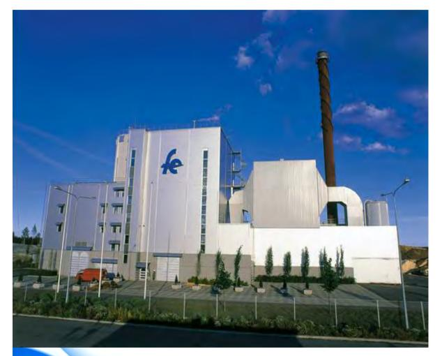
Forssan Energia Oy Fluidized bubbling bed Peat and wood fired Power 66 MW (thermal)
