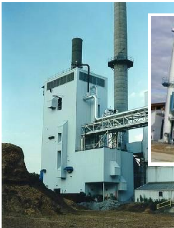
Rentech, SilvaGas gasifier, Burlington (US), 40 MW th_biomass
