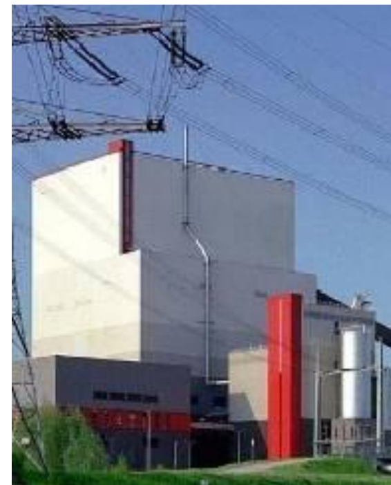
CFB (Lurgi), waste wood, Geertruidenberg (NL), co-firing PF boiler 85 MW th_biomass
