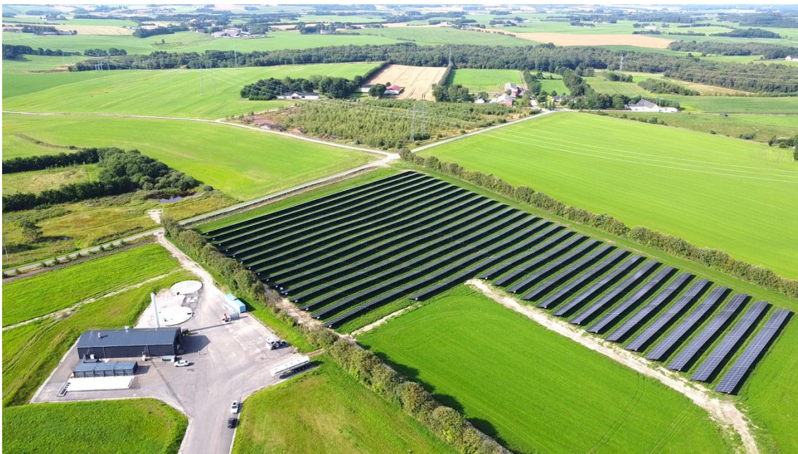
Figure 7 The biomass plant and newly added solar PVs at bird's view, photo credit: NORDEX FOOD
